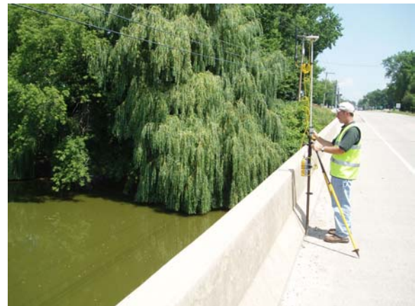
Surveying Upstream Water Levels
