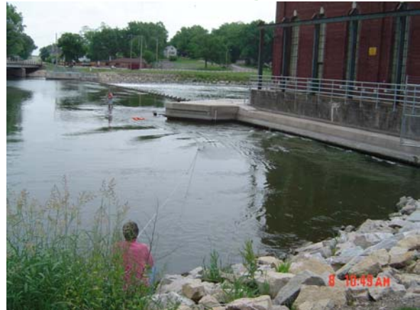
Measuring Flow Through Powerhouse
