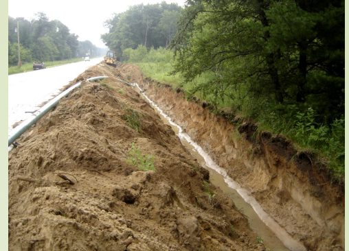
Typical trenching operations along state highway
