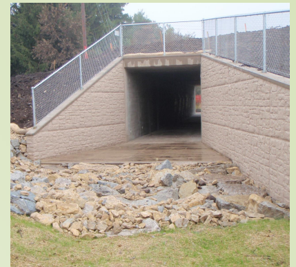
Constructed box culvert and portion of retaining wall
