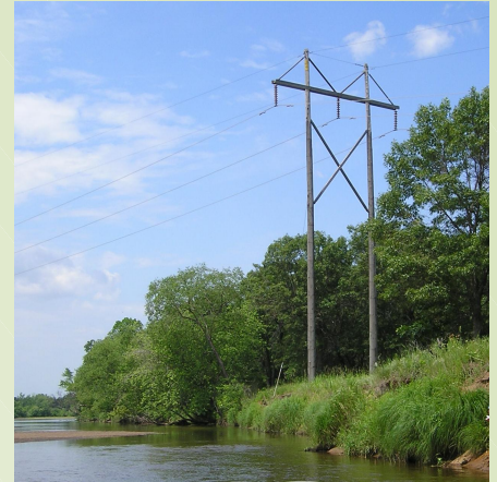
138 kV H-Frame Structure next to Wisconsin River Substation
